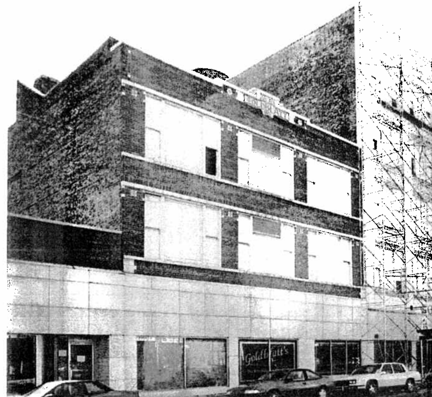
The oldest portion of Goldblatt's, at 1613-15 W. Chicago Ave., was built in 1921-22. Its three-story facade features ornamental brickwork, terra cotta details, and a pediment featuring the original Goldblatt's logo (above, left). The windows have been painted an off-white color. Top left: Architect Alfred Alschuler.
